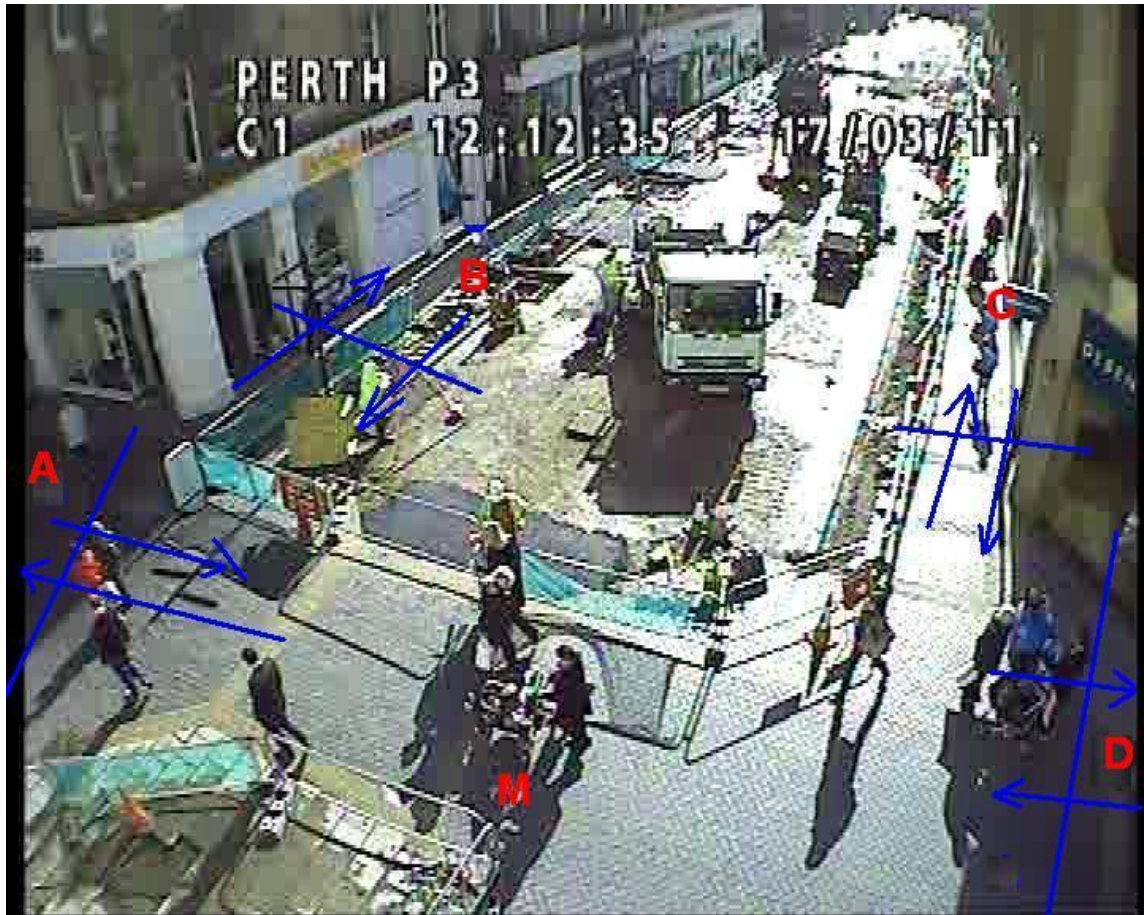
Figure 3.36 – Site P3 Pedestrian High Street – King Edward Street
